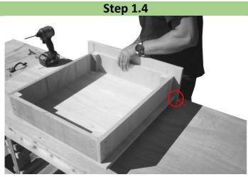
Place drawer front panel and make sure it is even spaced out on both sides. Secure with provided screws. **Repeat** steps 1 to 1.4 to complete rest of the drawers.
