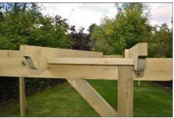
Place a second rafter on the main beam (slot side down) and use the supplied spacer to position it at correct distance from the end rafter. Repeat at the other end of the rafter
