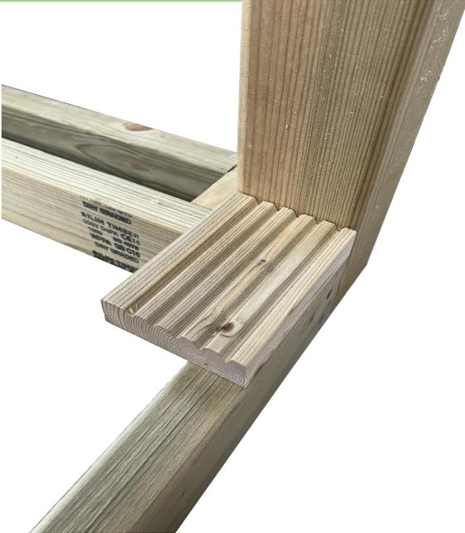
When your deck frame is finished, and the posts secured. Start placing your decking boards. First, add a narrower plank (pre-cut decking board) at the end of the decking frame, ensuring the edge is aligned with the decking frame.
