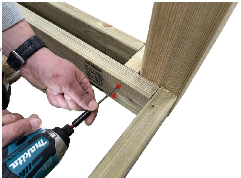
Secure the insert with two longer wood screws on both ends. Repeat this step for both sides.
