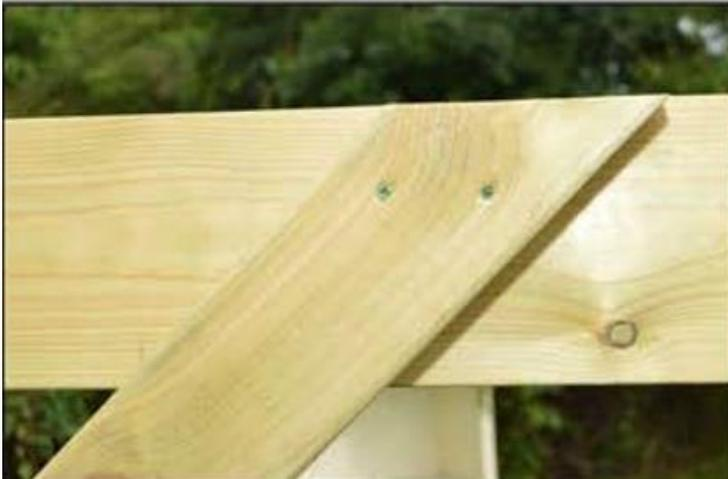
Make sure that brace is aligned with top of the rafter and bottom of the brace is central and flush with the upright. Secure using 2x 65mm screws at the top and 1x 85mm screw at the bottom
