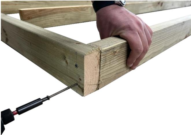
Secure the whole frame structure with provided longer wood screws.
