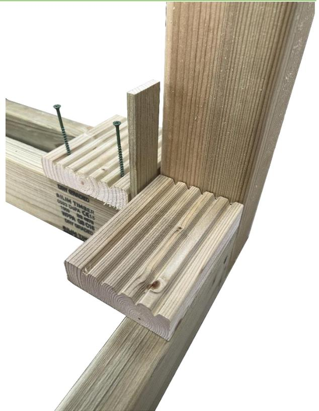
Lay out all the decking pieces across the infill joists and use a spacer block to evenly space them out. Secure the decking board with shorter wood screws. Important: the first and the last decking boards should be the same size.
