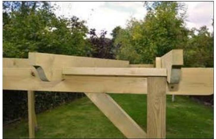
Place a second rafter on the main beam (slot side down) and use the supplied spacer to position it at correct distance from the end rafter. Repeat at the other end of the rafter
