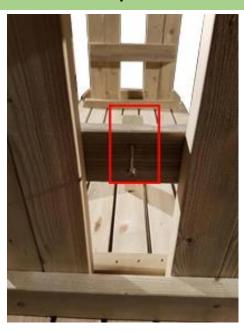
Ensure that the brace is lined up centrally on the table and attach it to the frame with a coach screw. Repeat steps to complete other side.
