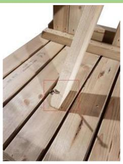
Place a cross brace in position as shown, ensuring that it is flush with the underside of the table frame and leg frame.
