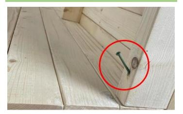
Don't forget to secure the back panel from the front via pre-drilled pilot holes with the provided 80mm screws.
