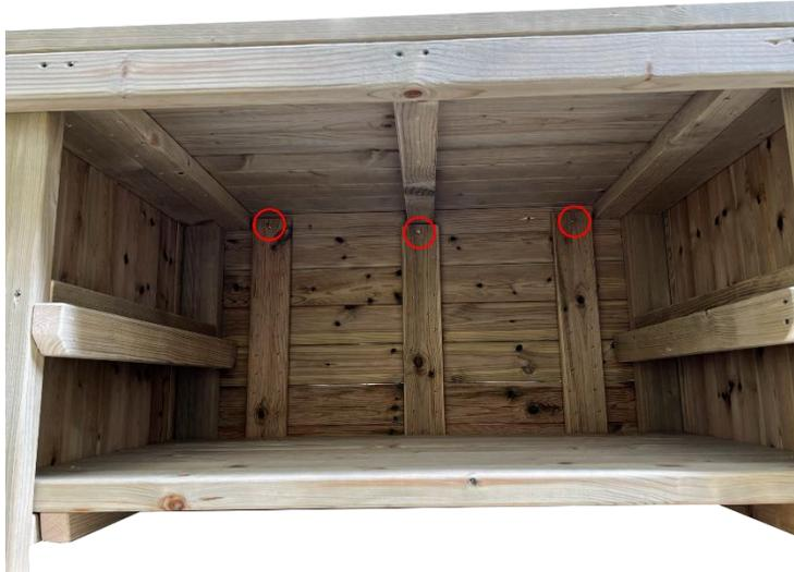
From the inside of the table, you will find 3x more guide holes where you need to secure the back panel to your assembly using the provided wood screws.
