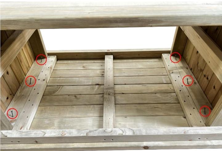
Secure the assembly to the worktop using 6x 60mm woodscrew through the guide holes.
