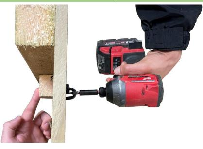
Fit the hook to the opposite side of the doors from the hinges to whichever height is the best for you with 2x black screws. Don't forget to attach the provided batten to the other side of the doors while screwing in the black screws to hide the pointy screw end's sticking out of doors.
