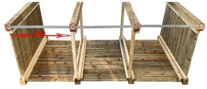
Now take the front bar and secure it with the 60mm screws as shown in the picture. Please don't forget to use the space bar (70cm) between the posts to ensure that the gap is correct.
