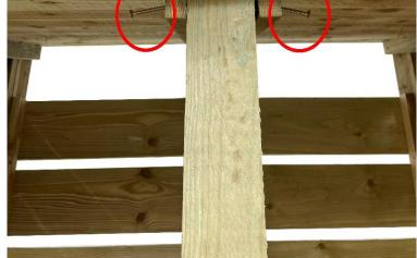
Ensure that both centre post sits flush with the roof's batten ends and is secure in place with 2 of the 65mm screws.
