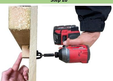
Fit the hook to the opposite side of the doors from the hinges to whichever height is the best for you with 2x black screws. Don't forget to attach the provided batten to the other side of the doors while screwing in the black screws to hide the pointy screw end's sticking out of doors.
