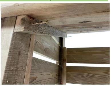
Check that the batten ends sit flush with the posts as shown. Now attach the roof to each end panel post with 65mm screws. Secure the rear of the roof using provided screws as well.
