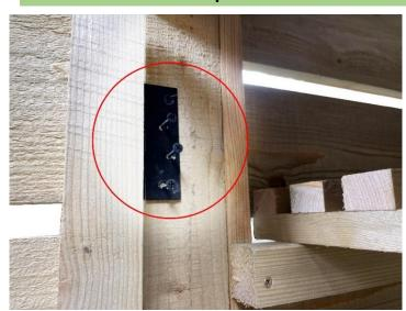
Align the top hinge in place, ensuring that the gap between the door and post is consistent at the top and bottom, then secure the top hinge in place using more of the black hinge screws.
