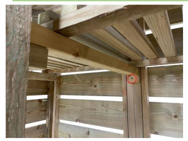
Place the kindling shelf on the braces and attach two last middle support braces in the middle between the front and back central posts using the provided screws, ensuring that the kindling shelf sits at the same level.
