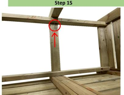
After ensuring that the gap at the bottom is the same as in the top, attach two of the centre posts to the base panel with the provided 80mm screws.
