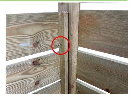
Using the 65mm screws provided, attach the batten on the back panel to the post of the end panel, ensuring that the batten remains vertically aligned to the post.
