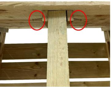
Ensure that the centre post sits flush with the roof's batten ends and is secure in place with 2 of the 65mm screws.
