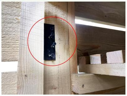
Align the top hinge in place, ensuring that the gap between the door and post is consistent at the top and bottom, then secure the top hinge in place using more of the black hinge screws.
