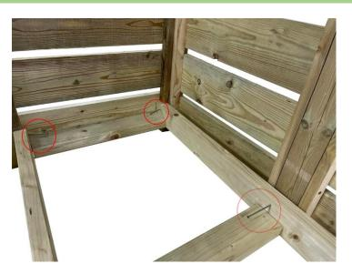
Remove the blocks from beneath the 2nd panel and then slide the base into position as shown, ensuring that the centre post and the central cross member of the base are aligned in the middle of the back assembly. Secure the base with the provided 85mm screws, just as shown in the picture.
