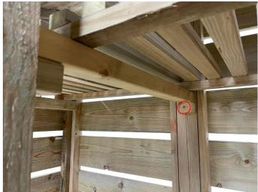
Place the kindling shelf on the braces and attach the last support brace in the middle between the front and back central posts using the provided screws, making sure that the kindling shelf sits at the same level.
