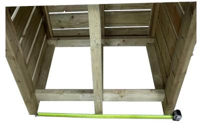
Fit the central post in the middle of the log store, measure the gaps, and ensure they are equal before securing the post with the screws.
