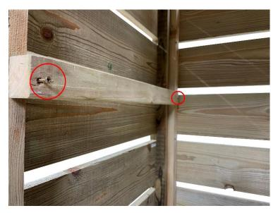
Please attach the side braces at your required height, secure it with the provided screws and lay the lattice section on top (If you don't have the kindling shelf, please skip this step.)
