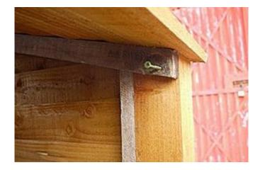
Check that the front batten ends sit flush with the posts as shown. Now attach the roof to each end panel post with 65mm screws.
