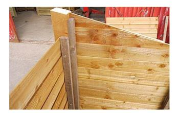
Secure the right side panel in place with 65mm screws.
