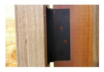
Align the top hinge in place, ensuring that the gap between the door and post is consistent at top and bottom then secure the top hinge in place using more of the black hinge screws.
