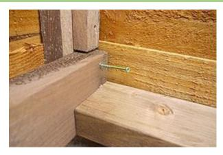
Now attach the base to the end panel rear posts, again using 1 of the 85mm screws for each side.
