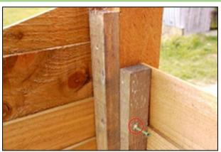
Using the 65mm screws provided, attach the batten on the side panel to the post of the end panel, ensuring that the batten remains vertically aligned to the post.
