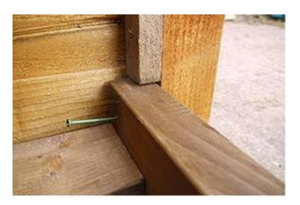
Attach the base to the end panel front posts using 1 of the 85mm screws for each side.
