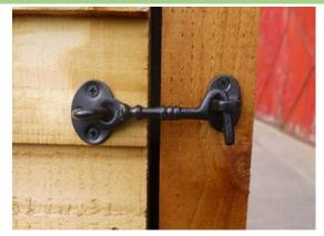
To fit the latch keeper plate, shut the door and hold the latch in the horizontal position. Now fit the keeper and mark its correct fixing position on the post using a pencil or bradawl before securing it in place using the screws provided.
