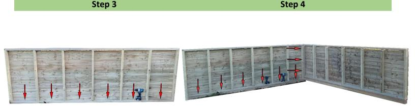
Take first half of the back panel which is marked **B1** and fit in on the longer slide securing it with the 6x 70mm coach screws.
