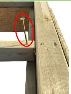
Secure each rafter end with a 1x120mm wood screw via predrilled pilot hole as shown in the picture. (2x 120mm wood screws per rafter.)
