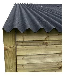
Place the roof panels on top of your assembly leaving 5cm sticking at the back and 10 cm sticking at the front
