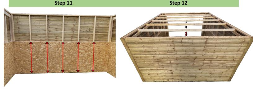
After making sure that all corpus panels are safe and secured with the necessary wood screws you can go and put on the kickboards in their places. Each OSB board will have its own marking which will show to which position it must go (**Front – Back – Sides**). Secure the kickboard with the 40mm woodscrews.
