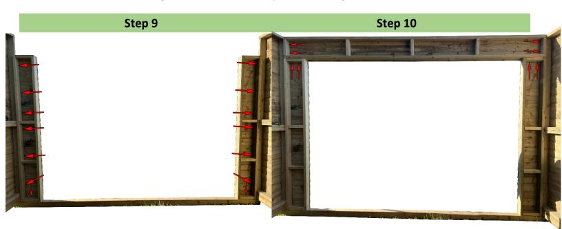
Place the front panels **FR** and **FL** as shown in the picture make sure that every side is aligned and secure each panel with 4x 70mm coach screws.
