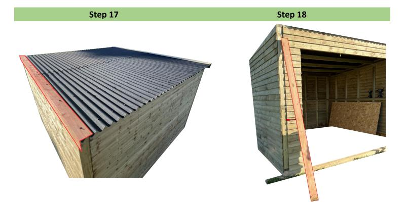
After screwing the whole roof into place, put the corners on your assembly, secure it from the sides with the 8x 40mm screws and from the top use 8x 80mm screws together with the caps, make sure that the corners are aligned with the roof ends.
