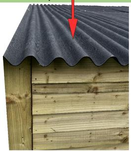
Use the provided screws with caps to secure the roof, start putting screws from the very first wave into the waves bump marked position.
