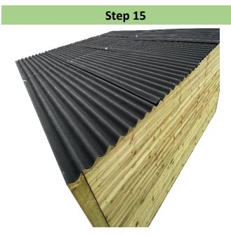
Keep putting on the rest of the roof panels making sure that the last roof wave would go underneath the new roof wave so that they could have a connection point. Step 16
