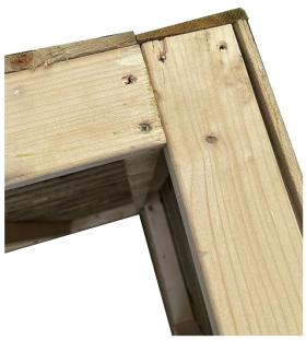
Take the side panel and secure it to the back panel with the 4x80mm wood screws via predrilled pilot holes.
