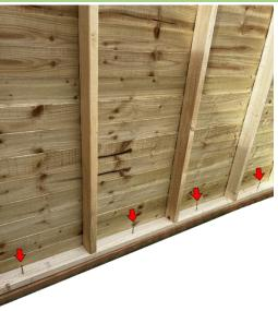
Now take 6x80mm wood screws and secure the back panel to the slides as shown in the picture.
