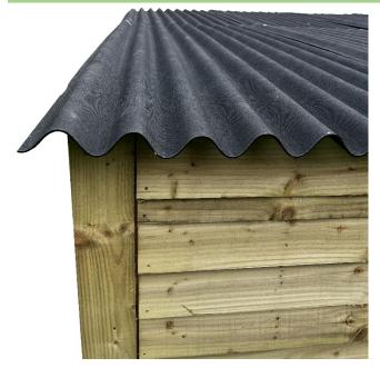
Place the roof on top of your assembly leave 5cm from front back and the sticking corner so that everything would spread equally.
