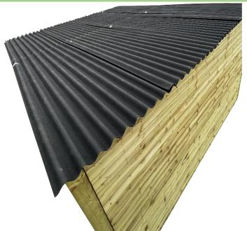
Keep putting on the rest of the roof panels making sure that the last roof wave would go underneath the new roof wave so that they could connect and be screwed per one screw. Please use the provided screws to secure the roof to the assembly.
