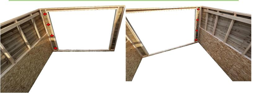
Place the front panel in the same manner and secure it with the 4x80mm wood screws making sure that everything is aligned.
