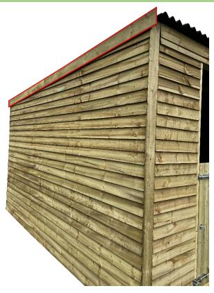
Place the second half of the cover aligning it with the first one. Again, secure it with the 16x40mm wood screws. Complete step 20 on the other side of the shelter as well.
