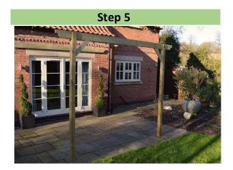
Carefully lift the completed structure into the upright position as shown and position in its final location before securing into place.
