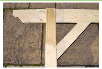
Place 500mm brace (standard or sculpted) as shown, align it so that its ends are flat and central against the runner and post.
