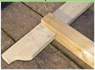
Now slide one of the runners and secure it with provided screws. Please note both sides of the runner must have the overhang of 40.5 cm.
