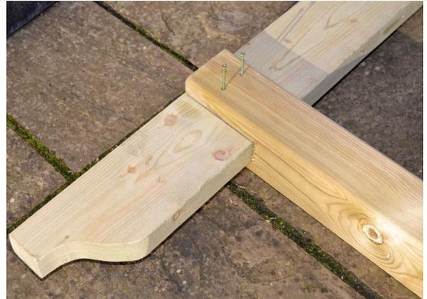
Now slide one of the runners and secure it with provided screws. **Please note both sides of the runner must have the overhang of 40.5 cm.**
