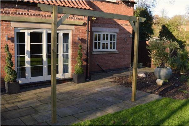
Carefully lift the completed structure into the upright position as shown and position in its final location before securing into place.
