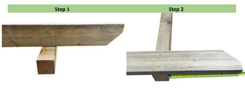
Take one of the posts and one of the runners and arrange on the floor as shown. Align the post to the marked pencil lines on the runner. Please note both sides of the runner must have an overhang of 41cm.
