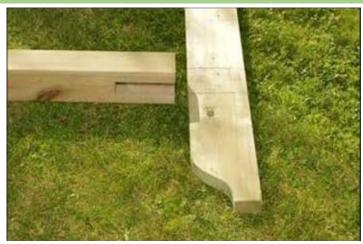
Put the upright perpendicular to the runner and its outside edge make sure it is aligned with the pencil mark near the runner's end
