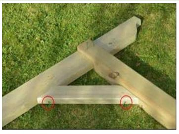
Then align one of the short braces as shown, make sure ends are flush and central against the main beam and upright. Secure it into place with 85mm screws use pre-drilled holes. Repeat steps 1-3 for the remaining 3 uprights and main beam
