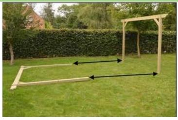
4.8m x 4.8m garden pergola kit version will have additional upright midway. Align uprights using pencil mark and secure with 85mm screws using pre-drilled holes. Then, attached short braces as shown in the picture and secure it with 85mm screws
