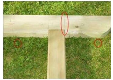
Slide the upright onto the main beam and fix into place using 2x 65mm screws through pre-drilled holes in the upright. Please note both sides of the runner must have an overhang of 40.5 cm.
