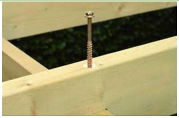
Now secure the correctly positioned rafter in using a coach screw through the pre-drilled hole on the top of the main beam and both end of the rafter.
