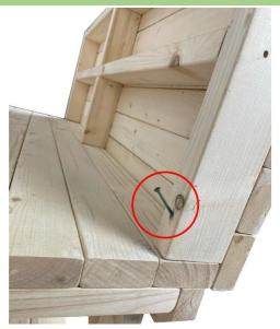
Secure the back panel via pre-drilled pilot holes with the 85mm screws just as shown in the picture.
