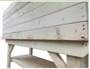
If you order version with back panel. Lift the back section into place. Ideally this will need to be held in place by a second person. Secure the back using the screws supplied.
