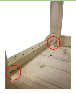
After making sure that the legs are pushed in the corners secure it with the provided screws just as shown in the picture.
