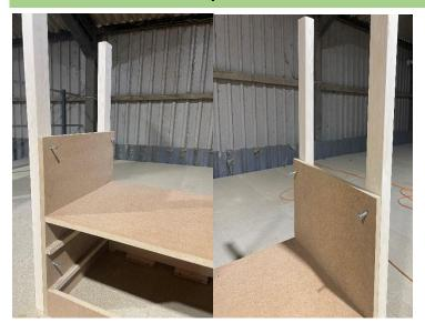
Before fixing the legs, please make sure that you are fixing workbench legs in the correct places please see numbers on the legs and match it with the numbers on the panels. After sorting the legs out, secure them with the confirmat screws, as shown in the picture.
