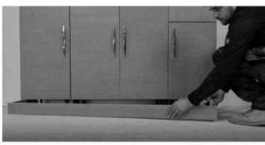
Secure both panels using confirmat screws. Repeat steps for the other side.
