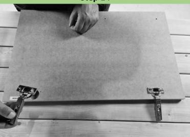
Now take your door (1x AGS4\_5). Place hinges into pre-drilled holes and secure with wood screws 4x16mm. Repeat this step for all three doors.
