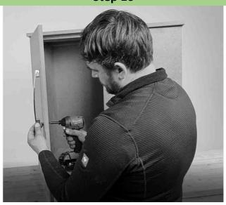
Now, using pre-drilled guide holes secure cabinet handles.
