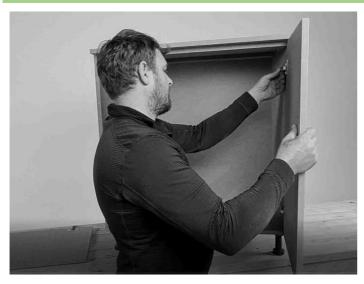
At this stage, take first door (AGS3\_5) and secure it into position as shown in the picture. Then take second door (AGS3\_5) and secure into position.
