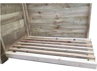
Drop the base into the slot in the side panel.
