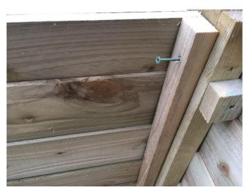
Line up the front panel and secure using the supplied screws through the pre-drilled holes.
