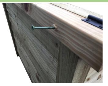
Secure the back roof rail using the supplied screws through the pre-drilled holes.
