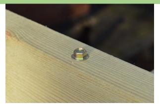
Fix the first rafter into place with a coach screw down through the top face into the wall plate and the end frame. Repeat steps 5 to 7 for the second outside rafter.
