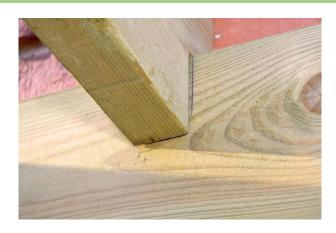
Make sure that the other end is aligned between the pencil marks on the wall plate. If necessary, adjust the position of the end frame to get everything square and properly positioned.
