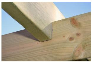
Continue adding the remaining rafters, use provided spacer to measure correct distance in between. Repeat this step until all the rafters are in place.
