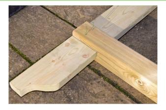
Now slot the remaining runner into the top of the post as shown using the pencil mark to align the runner with the outer edge of the post.
