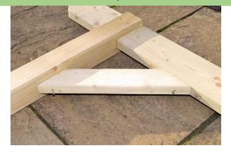
Fix the post into place on the runner using 2 x longer wood screws and then affix the diagonal brace using 2 x shorter screws as shown. Repeat steps 4 to 7 for other end of upright.
