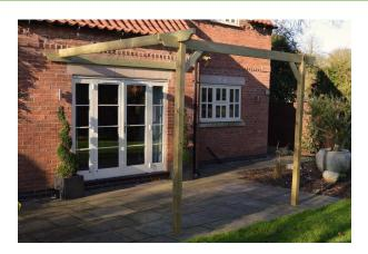
Now slot the first rafter in place so that it sits on the outside edge and butted to the post as shown.
