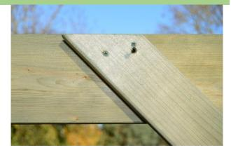
Now, add the longer braces (800mm) to the frame. Align top with the top edge of the rafter. Make sure that, bottom face of the brace is flush to the post. Secure with provide shorter wood screws. Repeat this step for both sides.
