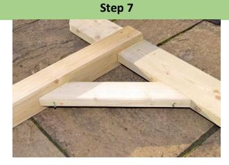
Fix the post into place on the runner using 2 x longer wood screws and then affix the diagonal brace using 2 x shorter screws as shown. Repeat steps 4 to 7 for other end of upright.
