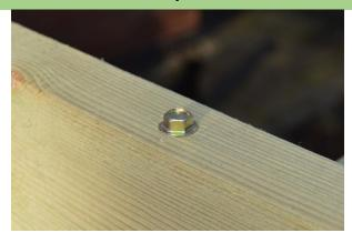
Fix the first rafter into place with a coach screw down through the top face into the wall plate and the end frame. Repeat steps 5 to 7 for the second outside rafter.
