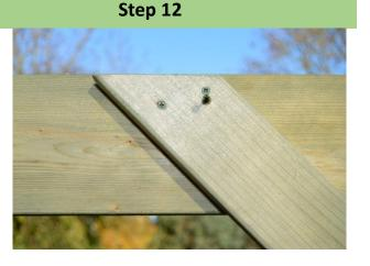
Now, add the longer braces (800mm) to the frame. Align top with the top edge of the rafter. Make sure that, bottom face of the brace is flush to the post. Secure with provide shorter wood screws. Repeat this step for both sides.
