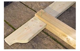
Now slot the remaining runner into the top of the post as shown using the pencil mark to align the runner with the outer edge of the post. **Please note both sides of the runner must have the overhang of 40.5 cm.**
