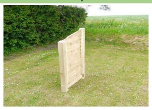
Stand the left-hand end panel (or right hand for the reversed roof version) upright on a flat, level surface.
