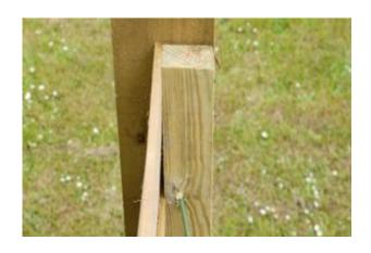
Attach the panel to the post by screwing through the batten using 65mm screws as before.
