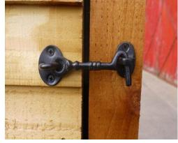
To fit the latch keeper plate, shut the door and hold the latch in the horizontal position. Now fit the keeper and mark its correct fixing position on the post using a pencil or bradawl before securing it in place using the screws provided.
