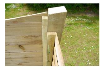
Using the 65mm screws provided, attach the batten on the back panel to the post of the end panel, ensuring that the batten remains vertically aligned to the post.
