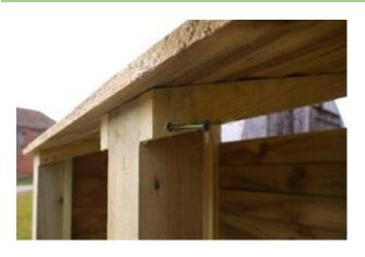
Make sure that the centre post sits flush with the roofs batten ends and secure in place with 1 of the 65mm screws.
