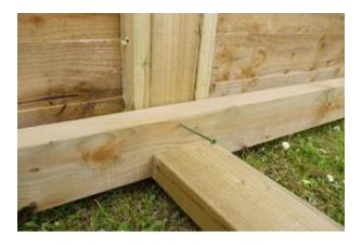
Using more of the 85mm screws now attach the base to the rear posts as shown.
