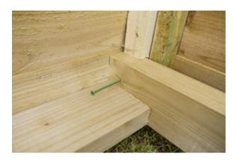
Now attach the base to the end panel rear post using one more 85mm screws
