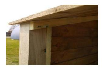
Carefully place the roof on top of the end panel posts ensuring that the batten ends sit flush with the posts as shown. Now attach the roof to each end panel post with 65mm screws.
