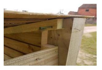
Secure the rear of the roof using 65mm screws as shown.
