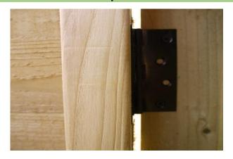
Secure the top hinge in place using more of the black hinge screws. Repeat steps 20 - 22 for any further doors as required.
