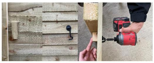
Fit the hook to the opposite side of the doors from the hinges to whichever height is the best for you with 2x black screws. Don't forget to attach the provided batten to the other side of the doors while screwing in the black screws to hide the pointy screw end's sticking out of the doors.
