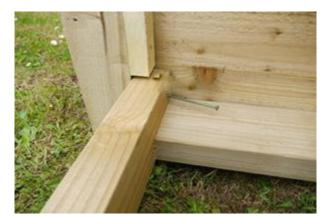
Attach the base to the end panel front post first, using 1 of the 85mm screw and then secure the rear post in the same way.
