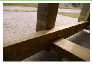
After making sure that the gap at the bottom is the same as in the top attach the centre post to the base panel with the provided 1x 80mm screw.
