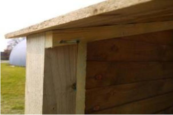
Check that the batten ends sit flush with the posts as shown. Now attach the roof to each end panel post with 65mm screws.
