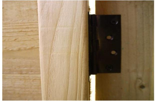
Secure the top hinge in place using more of the black hinge screws. Repeat steps 20 - 22 for any further doors as required.
