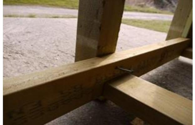
After making sure that the gap at the bottom is the same as in the top attach the centre post to the base panel with the provided 1x 80mm screw.
