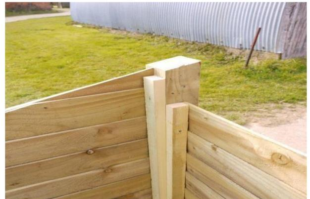
Using the 65mm screws provided, attach the batten on the back panel to the post of the end panel, ensuring that the batten remains vertically aligned to the post.
