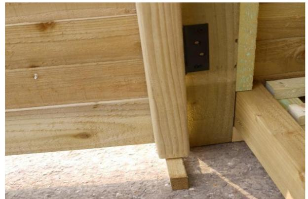
Place a spacer block at the front of the log store adjacent to the front-end post and rest the hinge side of the appropriate door on the block, aligning it vertically and horizontally for a good fit. Now use four of the supplied black hinge screws to affix the hinge to the post.
