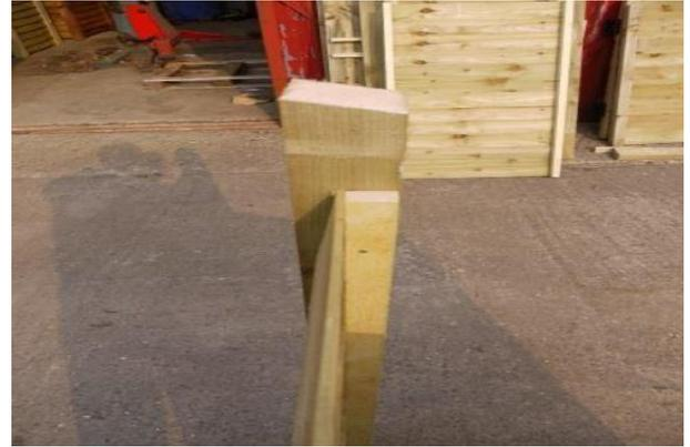
Attach the panel to the post by screwing through the batten using 65mm screws as before.
