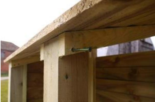
Make sure that the centre post sits flush with the roofs batten ends and secure in place with 1 of the 65mm screws.
