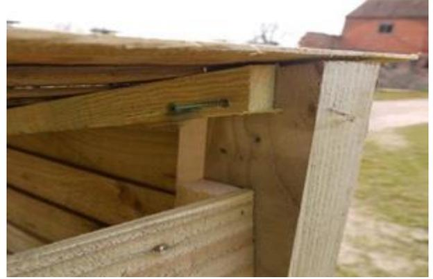
Secure the rear of the roof using 65mm screws as shown.
