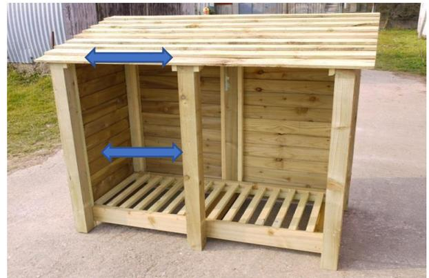
Fit a central post into the slotted roof position. By measuring the distance from the side panel to the central post and making sure it is equal at the bottom and the top. (**The space from the side panel to the central post must be equal to the back panels measurements**).
