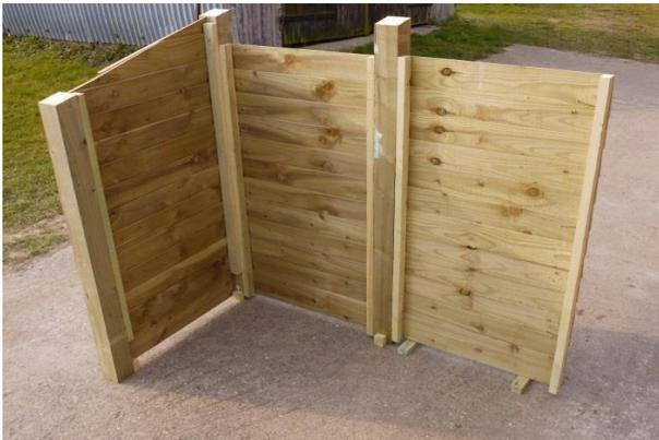
Rearrange the spacer blocks and offer up the next panel, aligning and attaching it as before.
