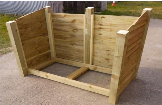
Slide the remaining end panel into place as shown above and attach it to the frame as you did with the first end panel with 85mm screws into the front and rear posts. If you are fitting a kindling shelf, omit steps 12 -14 and attach the front posts before fitting the kindling shelf & lattice and then attaching the roof.
