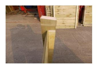
Attach the panel to the post by screwing through the batten using 65mm screws as before.
