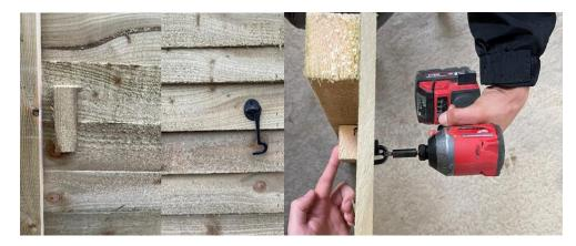
Fit the hook to the opposite side of the doors from the hinges to whichever height is the best for you with 2x black screws. Don't forget to attach the provided batten to the other side of the doors while screwing in the black screws to hide the pointy screw end's sticking out of the doors.
