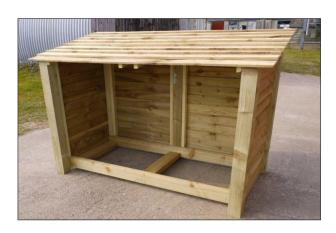
Carefully place the roof on top of the log store.
