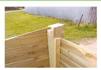
Using the 65mm screws provided, attach the batten on the back panel to the post of the end panel, ensuring that the batten remains vertically aligned to the post.
