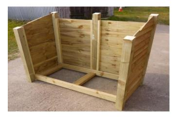
Slide the remaining end panel into place as shown above and attach it to the frame as you did with the first end panel with 85mm screws into the front and rear posts. If you are fitting a kindling shelf, omit steps 12 -14 and attach the front posts before fitting the kindling shelf & lattice and then attaching the roof.
