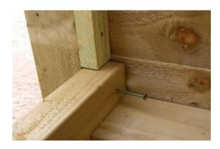
Attach the base to the end panel front post first, using 1 of the 85mm screw and then secure the rear post in the same way.
