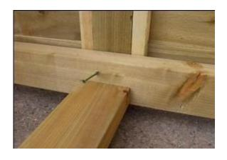
Using more of the 85mm screws now attach the base to the rear posts as shown.
