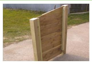
Stand the left-hand end panel (<u>or right hand for</u> <u>the reversed roof version</u>) upright on a flat, level surface.
