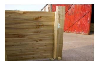
Align one of the longer posts (shorter for a reversed roof) with the other end of the back panel.
