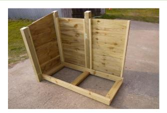
Remove the blocks from beneath the 2nd panel and then slide the base into position as shown, ensuring that the centre post and the central cross member of the base are aligned in the middle of the back assembly.
