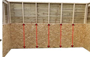
Now place both doors in their designated areas, spacing them out evenly. Secure door hinges to the shelter using 60mm woodscrews. After making sure that all corpus panels are safe and secured with the necessary wood screws you can go and put on the kickboards in their places. Each OSB board will have its own marking which will show to which position it must go (**Front – Back – Sides**). Secure the kickboard with the 40mm woodscrews.
