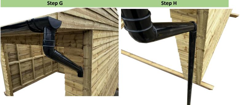
Attach one end of the longer pipe securely to the current structure, positioning it to face the shelter's front.
