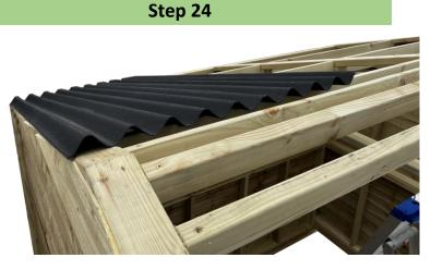
Note that the very top rafters should be positioned in the middle, aligning them with the centre of the shelter's roof.
