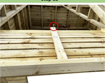
Between each of the roof panels, there is an additional predrilled hole. Insert a 70mm coach screw into these central predrilled holes. Fully tighten the coach screw to securely join the "F-L" and "F-R" panels to the shelter frame.
