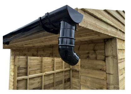
Fit one end of the pipe connection tube securely to the drainage system.
