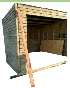
After everything is assembled and secured, take 4x provided featheredge boards and place them as shown in the picture hiding the connection points, leaving the thicker end of the board sticking outside and secure each featheredge plank with the provided nails.
