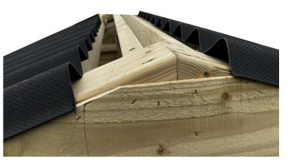
Keep putting on the rest of the roof panels making sure that the last roof wave would go underneath the new roof wave so that they could have a connection point.
