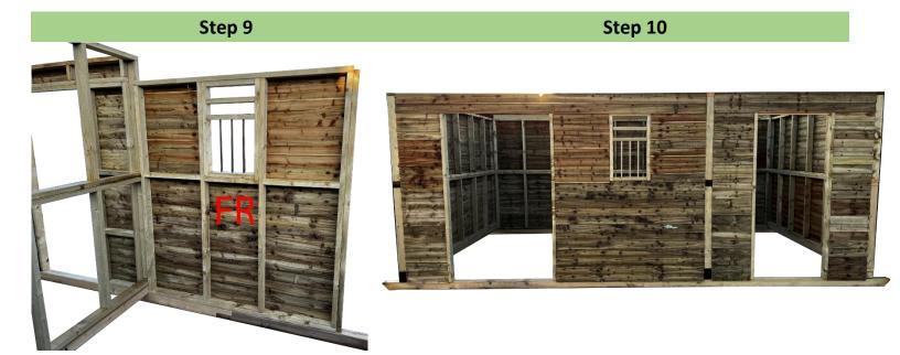
Proceed to install the rest of the panels into their located areas following the markings on the parts.
