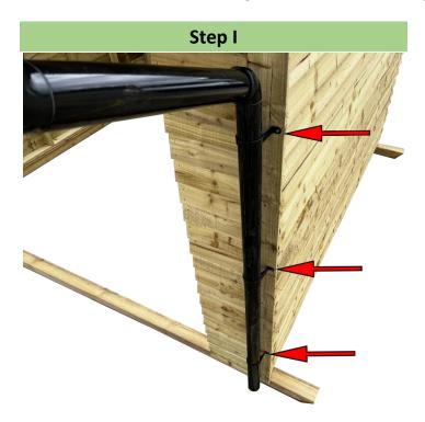
Securely attach the long pipe to the front edge of the shelter using the 3x provided pipe brackets. Insert the provided 40mm woodscrews through the predrilled holes on each bracket to firmly attach them to the shelter's structure.
