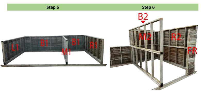
Follow the markings on the panels and secure all the remaining first-floor panels to their places in the same manner as previously through the provided pilot holes.
