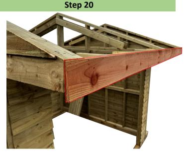
Position a featheredge board underneath the roof panels to complete the roof design. Secure the featheredge board in place using three 40mm wood screws.
