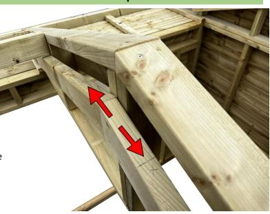
Identify the marked places on the highest point of the triangles, which indicate where the roof rafters should be aligned and secured.
