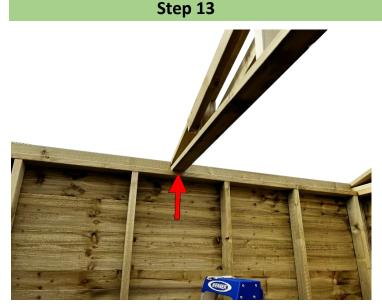
Locate the middle triangle labeled F-M. At the back of the shelter, you will find a designated cut-out area. Insert one end of the "F-M" triangle into this cut-out to secure it in place. Proceed to Step 15 at the front of the shelter, where you will find a marked place for aligning the front of the "F-M" triangle.
