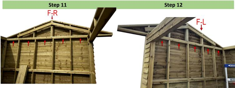
Position the roof structure triangle labelled "F-R" on the right side of the assembly as shown in the provided picture. Secure the triangle in place using the supplied 70mm coach screws. Insert the screws through the predrilled pilot holes located at the bottom of the structure, following the directional arrows in the diagram.
