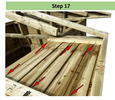
For each roof cover (both "F-L" and "F-R"), secure them in place using six 80mm wood screws. Insert the wood screws through the predrilled pilot holes located on each roof cover. Ensure the screws are tightened securely to firmly attach the roof covers to the shelter's structure.
