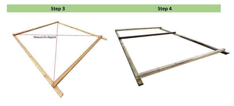
After securing all 4x corners measure both diagonals they must be the same length to continue your assembly.
