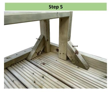
Following the leg's secure attachment, proceed to place 2x support braces as indicated in the provided illustration. Two support braces should be positioned on each leg. Once in place, secure the support braces firmly using the provided wood screws. Ensure the screws are tightened adequately to establish strong support and reinforce the overall structure.
