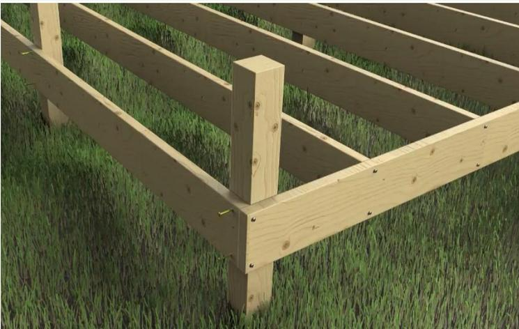
Secure the frame to the posts using the provided wood screws.
