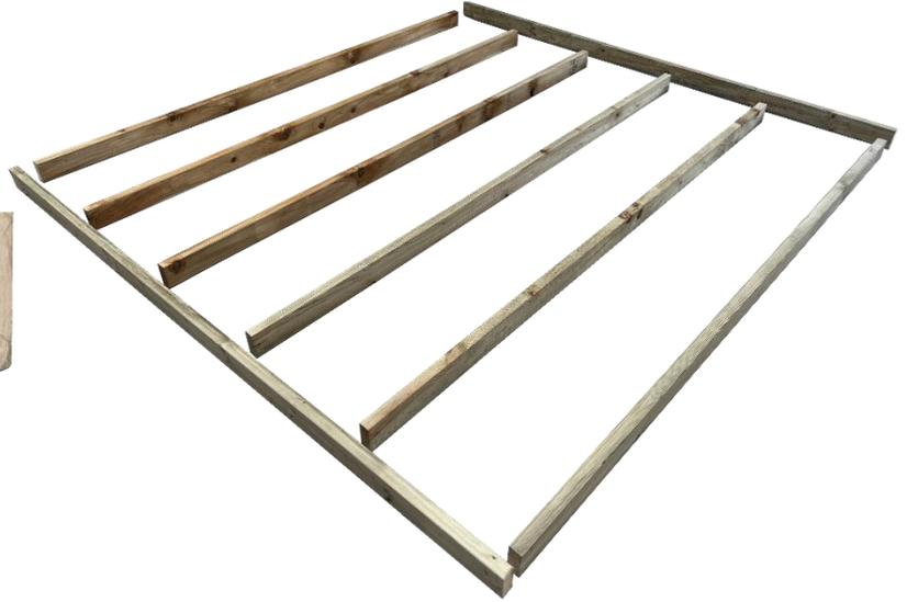
Ensure that the markings on the frame ends are facing inwards and that all the decking rafter slats are evenly spaced out and aligned with all the pencil lines.
