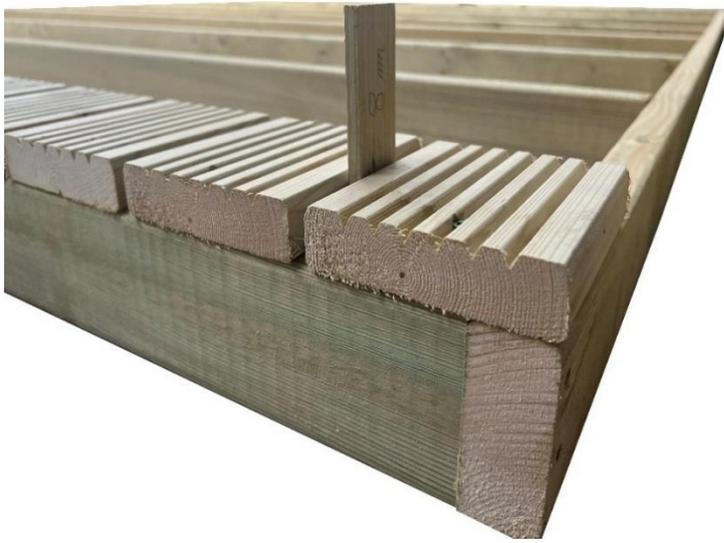
Lay the decking strips on the frame, running them across the joists. Space them out, **using the provided spacer** so they are evenly distributed and running parallel with one another. Fix each strip into place with 2 x wood screws down both edges and then wherever the decking strip meets a joist.
