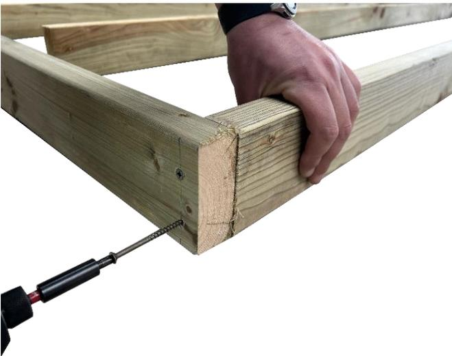
After all the joists are aligned secure each joist ends with 2x of the provided wood screws.
