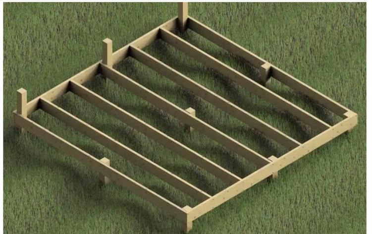
Once the frame is securely attached to the posts and you are satisfied that it is level, cut the post tops off flush with the frame as shown.
