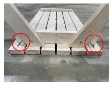
Now, using 2 of the supplied coach screws and the predrilled holes, secure the table A-frame to the fixing batten on the tabletop.
