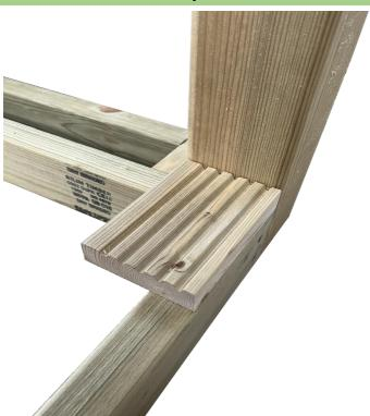
When your deck frame is finished, and the posts secured. Start placing your decking boards. First, add a narrower plank (pre-cut decking board) at the end of the decking frame, ensuring the edge is aligned with the decking frame.
