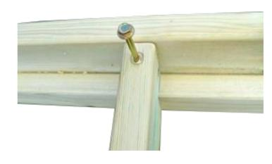
When the top pergola frame is completed and secured. Drop the rafters into place on the main beam and use a spacer bar to space out your rafters evenly. Use 100mm coach bolts to secure rafters on both sides.
