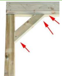
Then, align one of the short braces as shown (500mm). Align them to the underside of the batten on the main beam and the lower end to the corner post. Use shorter wood screws to secure the brace. Repeat this step for the braces.
