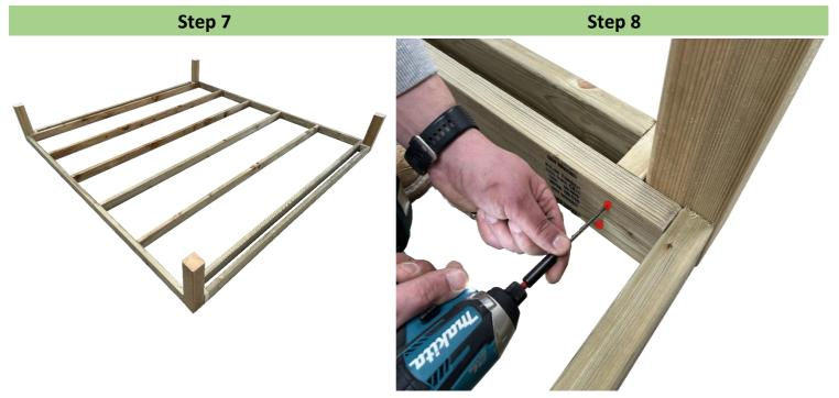
When all four posts are secured into place. Take pre-made front and back inserts for your frame kit and place them as shown in the picture.
