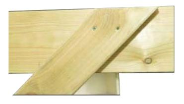
Now, align the long brace (700mm) with the top of the edge rafter and secure it via predrilled guide holes with shorter wood screws. Make sure that the bottom edge sits flush against the post.
