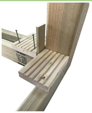
Lay out all the decking pieces across the infill joists and use a spacer block to evenly space them out. Secure the decking board with shorter wood screws.
