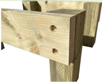
Align the edge rafters with the post ends and secure both sides with the two 100mm coach bolts. Repeat this step for the other post.
