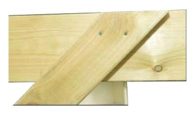
Now, align the long brace (700mm) with the top of the edge rafter and secure it via predrilled guide holes with wood screws. Make sure that the bottom edge sits against the post.
