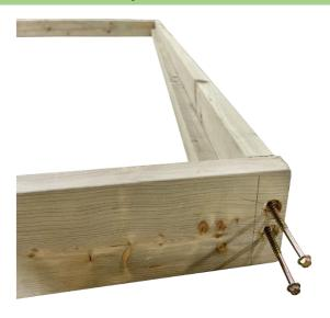
Take the edge rafter and, align it with the post ends, secure both sides with the two 100mm coach bolts. Repeat this step for the other post.
