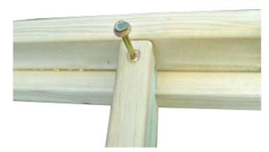
Working from within the structure you have assembled, use the supplied spacer to position your rafter second rafter at the correct distance from your edge rafter. Repeat at the other end of the rafter. Secure it with provided 100mm Coach screws.
