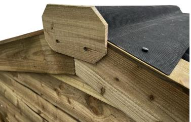
Place the middle roof covers in position, ensuring they are aligned in the middle of the shelter and effectively cover the previously empty gap. Secure each middle roof cover firmly using 80mm wood screws, together with the provided caps.
