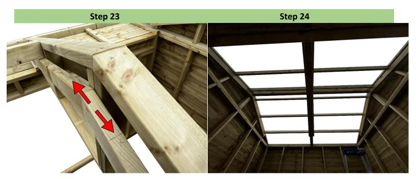
Identify the marked places on the highest point of the triangles, which indicate where the roof rafters should be aligned and secured.
