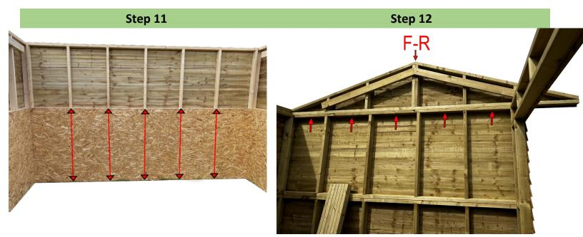
After making sure that all corpus panels are safe and secured with the necessary wood screws you can go and put on the kickboards in their places. Each OSB board will have its own marking which will show to which position it must go (Front – Back – Sides). Secure the kickboard with the 40mm woodscrews.
