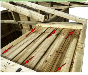
Take the two roof covers marked "F-L" and "F-R." Position the "F-L" roof cover on the left side of the roof, aligning it precisely as shown in the picture. Similarly, place the "F-R" roof cover on the right side of the roof, following the picture for accurate alignment. Ensure that both roof covers fit securely and cover the designated areas completely.
