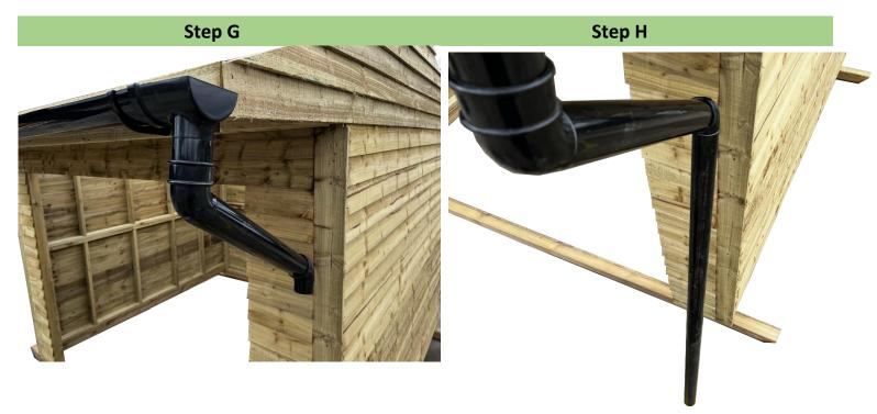
Attach one end of the longer pipe securely to the current structure, positioning it to face the shelter's front.
