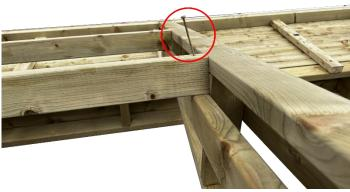
Take the roof front featheredge cover board. Align the pointy end of the cover board with the roof structure, as shown in the illustration or picture. Secure the board in place using 40mm wood screws.
