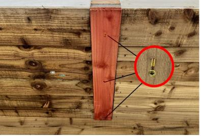
Between each of the roof panels, there is an additional predrilled hole. Insert a 70mm coach screw into these central predrilled holes. Fully tighten the coach screw to securely join the "F-L" and "F-R" panels to the shelter frame.
