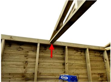
Locate the middle triangle labeled F-M. At the back of the shelter, you will find a designated cut-out area. Insert one end of the "F-M" triangle into this cut-out to secure it in place. Proceed to Step 15 at the front of the shelter, where you will find a marked place for aligning the front of the "F-M" triangle.
