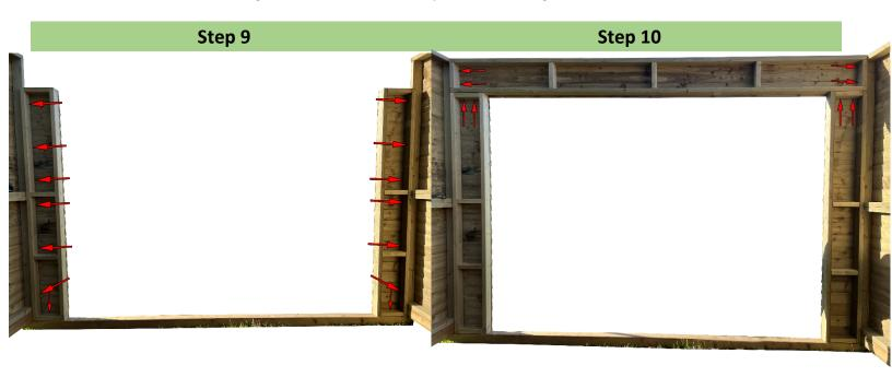
Place the front panels **FR** and **FL** as shown in the picture make sure that every side is aligned and secure each panel with 4x 70mm coach screws.
