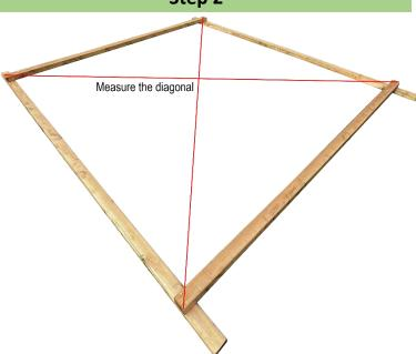
Take two of the smaller slides and place them on two of the longer slides as shown in the picture, before securing it with the coach screw or the metal corner make sure that the shorter slides are properly aligned with the marked line.
