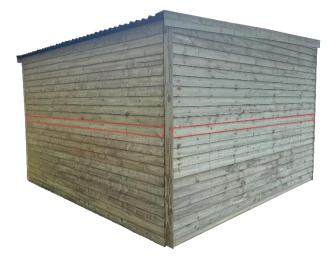
After everything is assembled and secured, take 4x provided featheredge boards and place them as shown in the picture hiding the connection points, leaving the thicker end of the board sticking outside and secure each featheredge plank with the provided nails.
