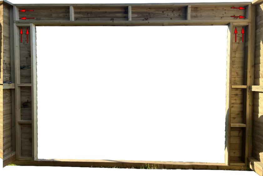
Place the front panels **FR** and **FL** as shown in the picture make sure that every side is aligned and secure each panel with 4x 70mm coach screws.
