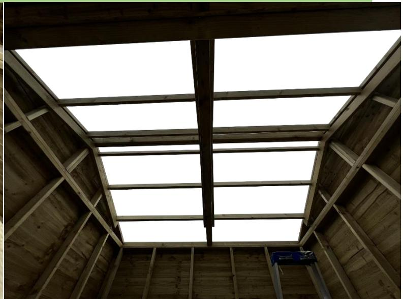
Note that the very top rafters should be positioned in the middle, aligning them with the centre of the shelter's roof.
