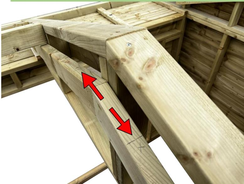
Identify the marked places on the highest point of the triangles, which indicate where the roof rafters should be aligned and secured.
