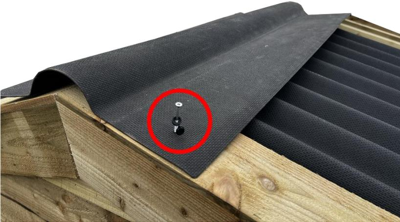
Place the middle roof covers in position, ensuring they are aligned in the middle of the shelter and effectively cover the previously empty gap. Secure each middle roof cover firmly using 80mm wood screws, together with the provided caps.
