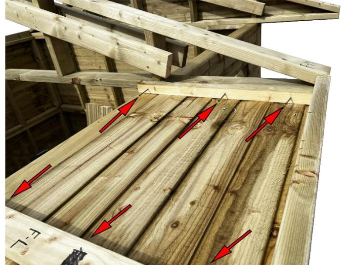
Take the two roof covers marked "F-L" and "F-R." Position the "F-L" roof cover on the left side of the roof, aligning it precisely as shown in the picture. Similarly, place the "F-R" roof cover on the right side of the roof, following the picture for accurate alignment. Ensure that both roof covers fit securely and cover the designated areas completely.
