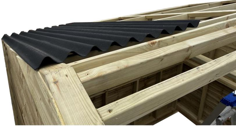
Position the roof panels on top of your assembly, ensuring they cover the entire shelter structure. Leave approximately 7cm (2.75 inches) of the roof panels protruding at both the back and front of the assembly. Use the provided screws with caps to secure the roof.
