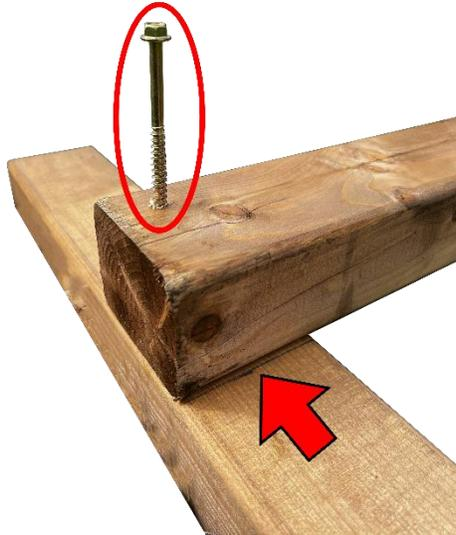
Take two of the smaller slides and place them on two of the longer slides as shown in the picture, before securing it with the coach screw or the metal corner make sure that the shorter slides are properly aligned with the marked line.
