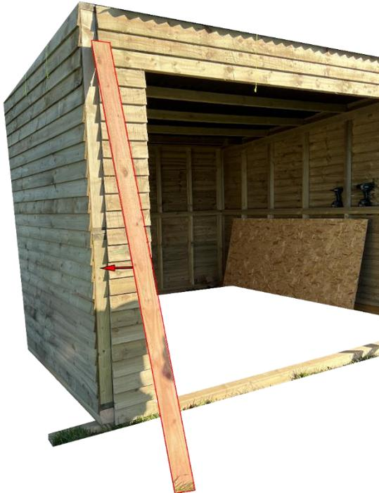
After everything is assembled and secured, take 4x provided featheredge boards and place them as shown in the picture hiding the connection points, leaving the thicker end of the board sticking outside and secure each featheredge plank with the provided nails.
