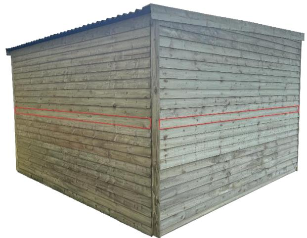
On each of the connection point, there will be one featheredge board which is not attached. Use the provided nails and secure each side of the building.
