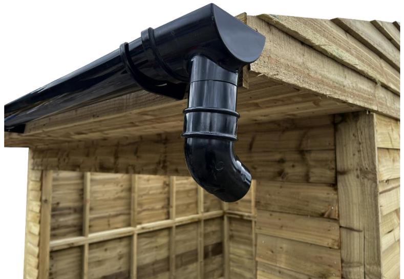
Take the provided elbow connection component. Attach the elbow connection to the previously fitted pipe connection tube securely.
