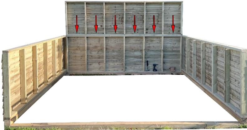
Now take the second half of the back panel **B2** and place it on top of the first securing it with the 6x 70mm coach screws as shown.
