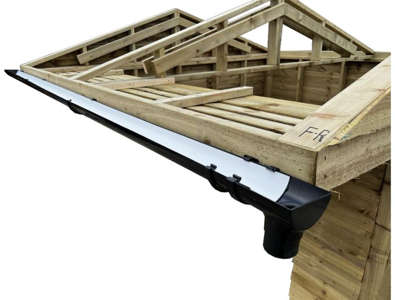
Take the assembled gutter pipe, which includes both ends securely attached with the appropriate fittings. Position the assembled gutter pipe along the previously fastened holders on the front edge of the shelter.
