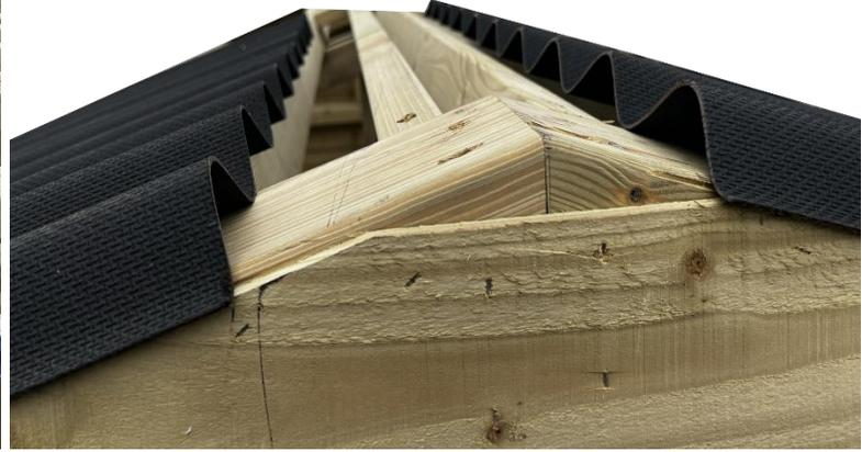
Keep putting on the rest of the roof panels making sure that the last roof wave would go underneath the new roof wave so that they could have a connection point.
