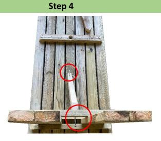
Place a cross brace in position as shown, ensuring that it is flush with the underside of the table frame and secure it with the provided coach screws.
