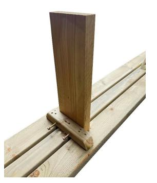
Measure the distance between the left and middle battens and then between the middle and right battens on the underside of the bench top, and place the third middle support leg, made from a 2x6 timber plank, in the middle of the larger gap, securing it with two of the provided coach screws.
