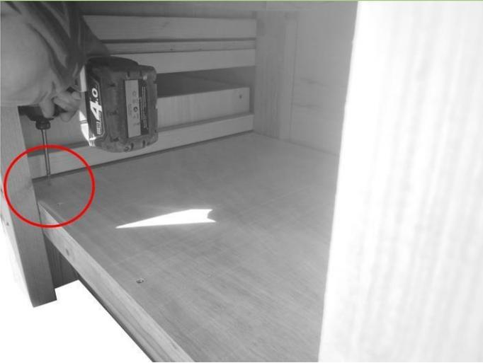
When you done assembling drawers, slide base shelf into position and secure with provided screws, repeat this step on the other side. **If you have double shelf option, repeat this step twice.**
