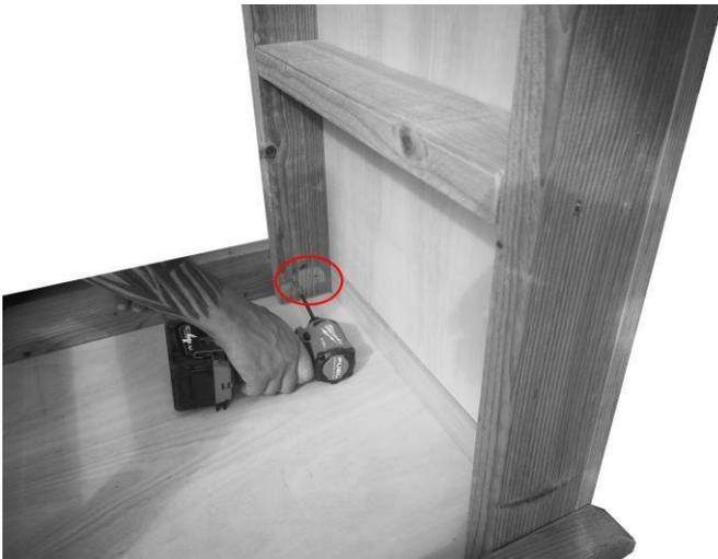
Secure with the supplied screws use pre-drilled guide holes.
