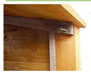
Check that the front batten ends sit flush with the posts as shown. Now attach the roof to each end panel post with 65mm screws.
