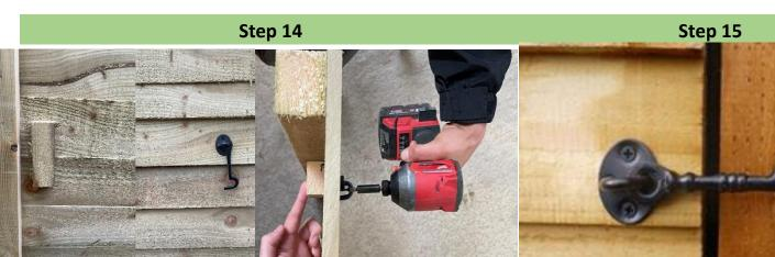
Fit the hook to the opposite side of the doors from the hinges to whichever height is the best for you with 2x black screws. Don't forget to attach the provided batten to the other side of the doors while screwing in the black screws to hide the pointy screw end's sticking out of the doors.
