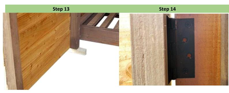
Place a spacer block at the front of the log store adjacent to the front-end post and rest the hinge side of the appropriate door on the block, aligning it vertically and horizontally for a good fit. Now use four of the supplied black hinge screws to affix the hinge to the post. Align the top hinge in place, ensuring that the gap between the door and post is consistent at top and bottom then secure the top hinge in place using more of the black hinge screws.
