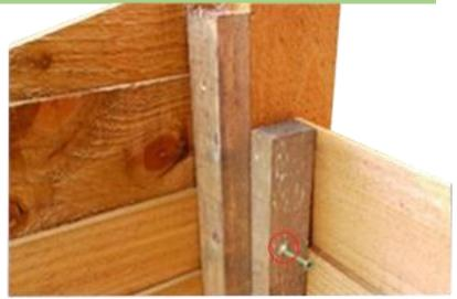
Arrange the 2 spacer blocks on the ground, adjacent to the side panel as shown in the photo above. Now place a back panel on the blocks, at 90° to the end panel, aligning the 2 panels ready for fixing.
