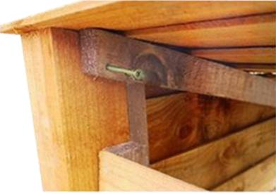
Secure the rear of the roof using 65mm screws as shown. Your log store is now complete. If your log store came with doors, proceed to step 13.
