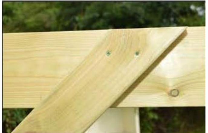
Make sure that brace is aligned with top of the rafter and bottom of the brace is central and flush with the upright. Secure using 2x 65mm screws at the top and 1x 85mm screw at the bottom
