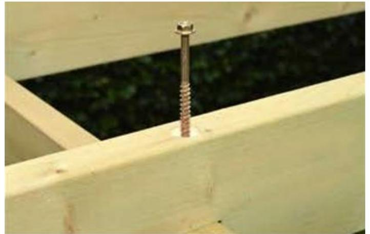
Now secure the correctly positioned rafter in using a coach screw through the pre-drilled hole on the top of the main beam and both end of the rafter.
