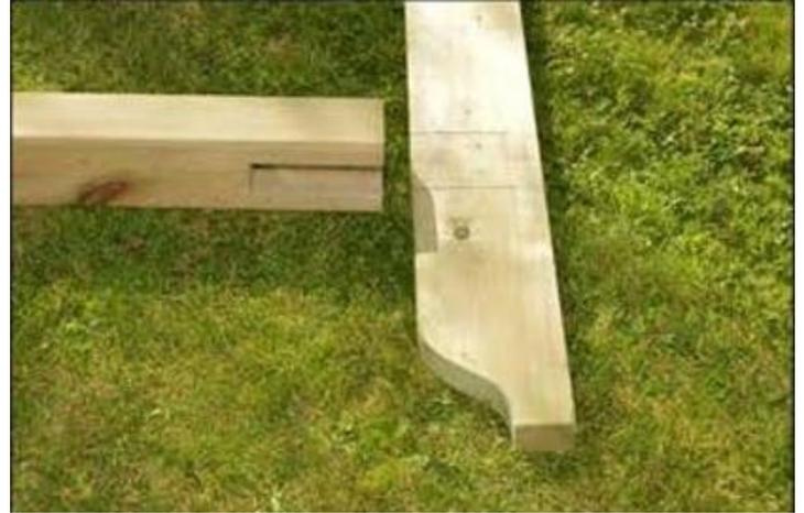
Put the upright perpendicular to the runner and its outside edge make sure it is aligned with the pencil mark near the runner's end
