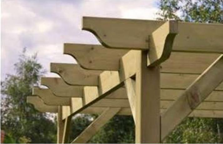
Continue adding and securing the remaining 3 rafters, using the spacer as before to ensure the correct spacing.
